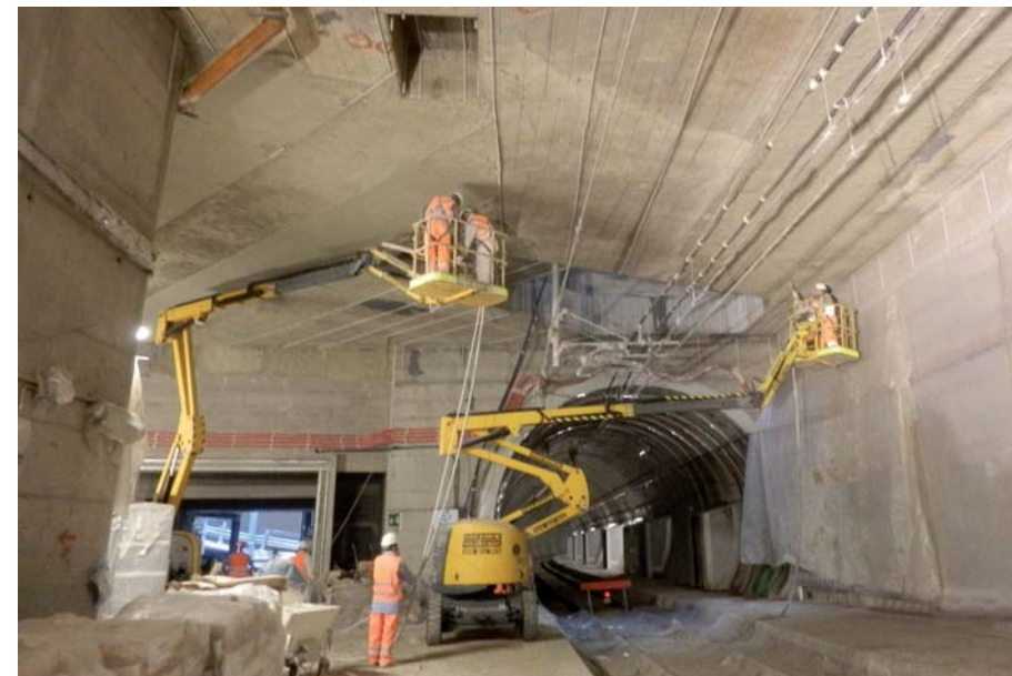
Securing tunnels with railway lines in service. (ITALFERR- RFI)
